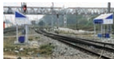
Solar powered Rolling In/Out huts, NFR
