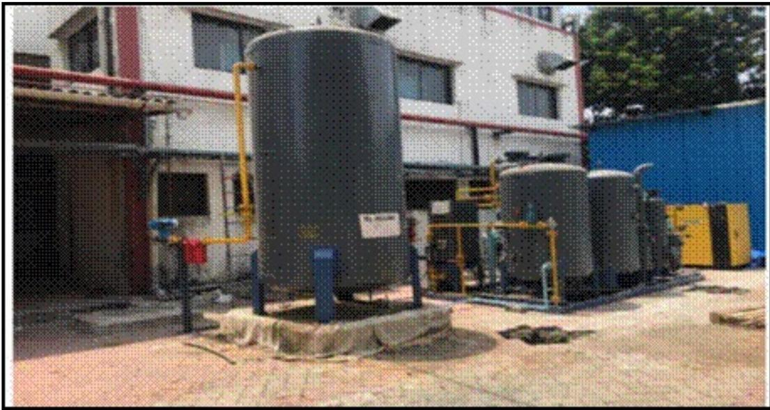
**Modified Nitrogen plant to generate medical Oxygen, installed by M/s. UPL Ltd. at L
